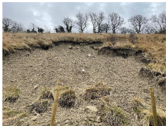
Figure 6: Close Up of landslip below horse
