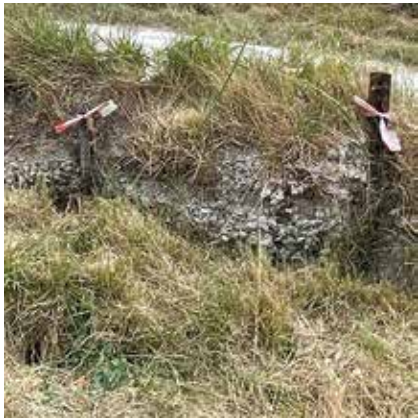
Fig 3: Face of 'new' revetment.
