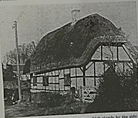
The 16th-century half-timbered cottage which stands by the side of Broad Town's main street. In the background can be seen the 100-year-old church.
